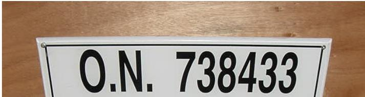
Example of documentation number permanently mounted on bulkhead
